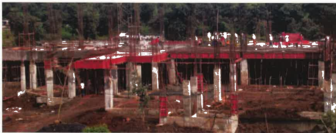
Library-cum-Computer Center under construction
