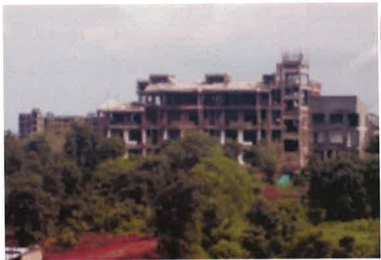
Visitors Hostel under construction
