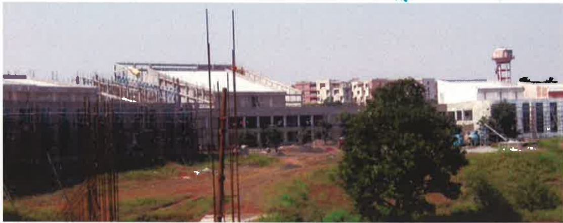
Lecture Hall and Tutorial Complex under construction
